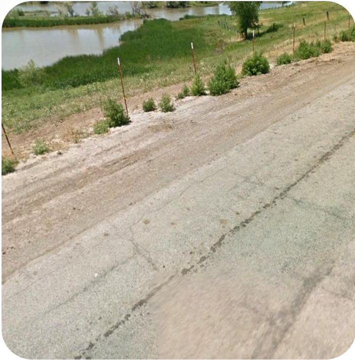
Looking southwest near 2425 West
